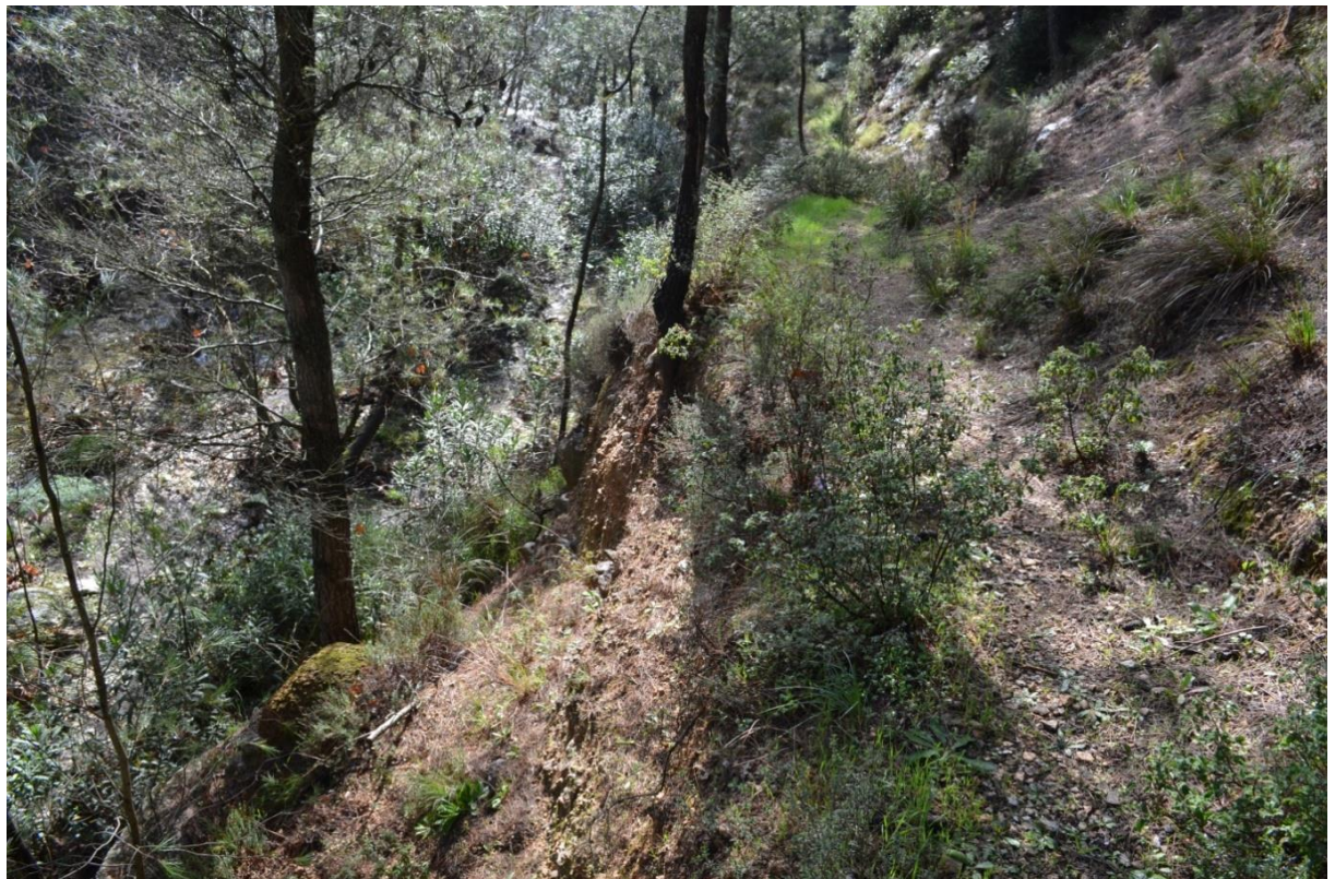
Figure 59. The road is badly ruined where the Janoula river (on the left) flows particularly close to the roadside. The road retaining wall has fallen down and the road bed itself is eroding. Photograph taken from north.
