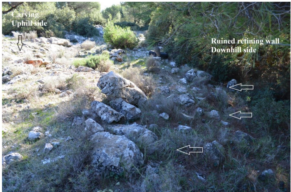
Figure 44. Badly preserved remnants of the road retaining wall (foreground and right), road surface (centre), and carving along the uphill side (upper left corner). Photograph taken from north.
