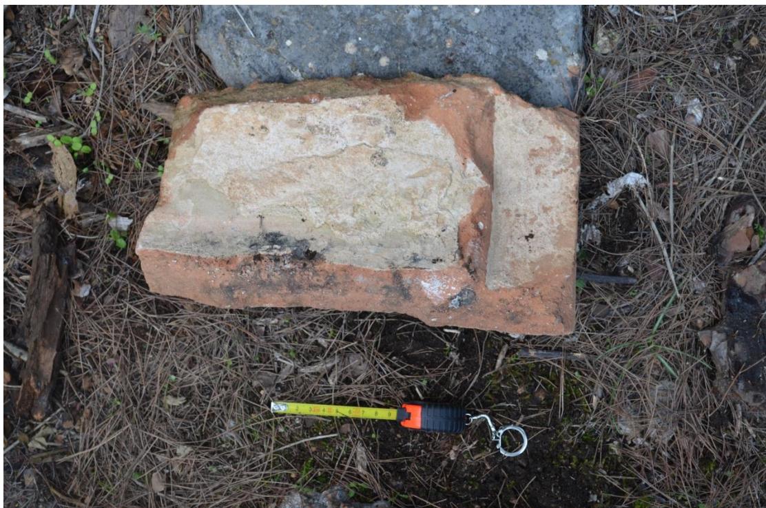
Figure 128. Large terracotta tile-like component; inner side with traces of mortar attached.
