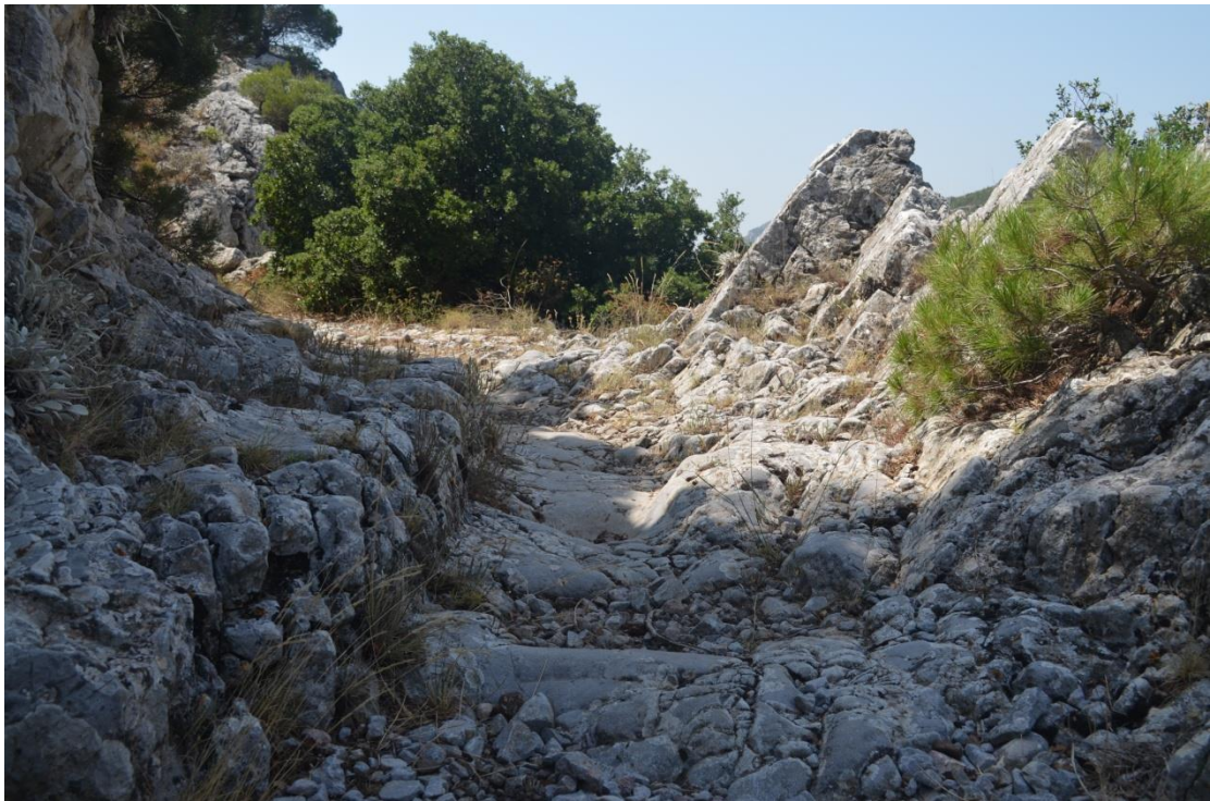
Figure 109. Carving cut in the central part of the road, differing from other sections that are cut closely against the uphill side. Photograph taken from north.
