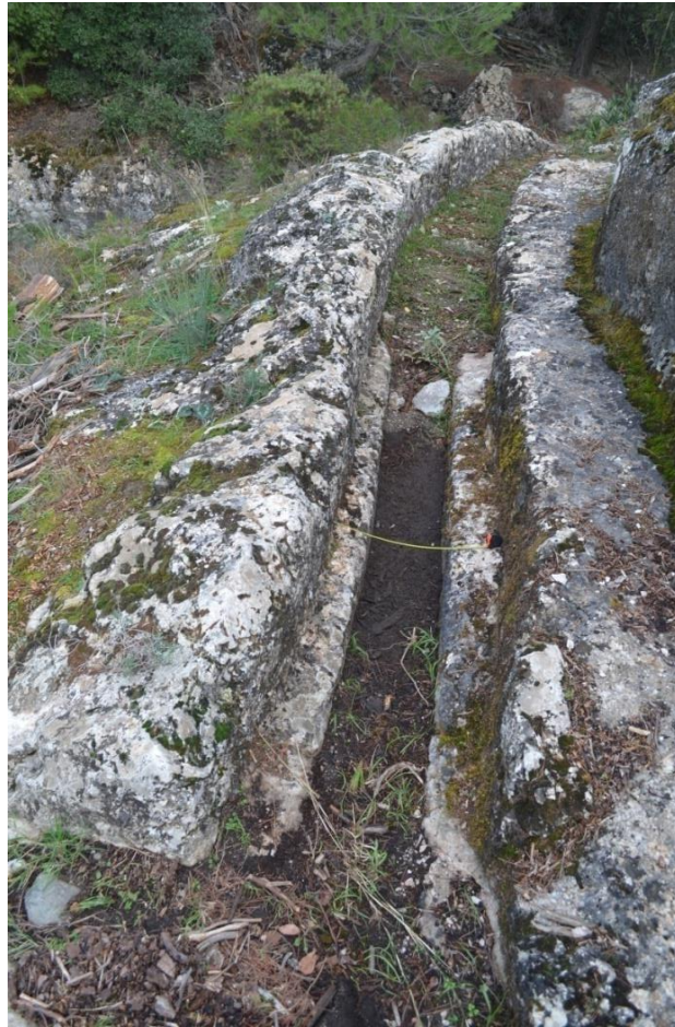
Figure 123. Ancient aqueduct deeply carved in the rock with chiseled flanks for accommodating cover slabs. Photograph taken from west.
