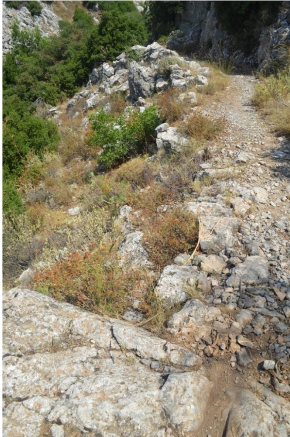
Figure 113. In certain parts the retaining wall collapsed leaving the road exposed to erosion. Photograph taken from south.
