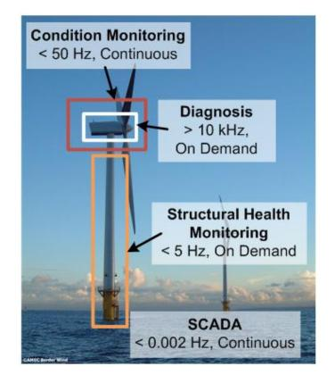
Figure 2.3: Monitoring systems on WT (Crabtree 2010).
