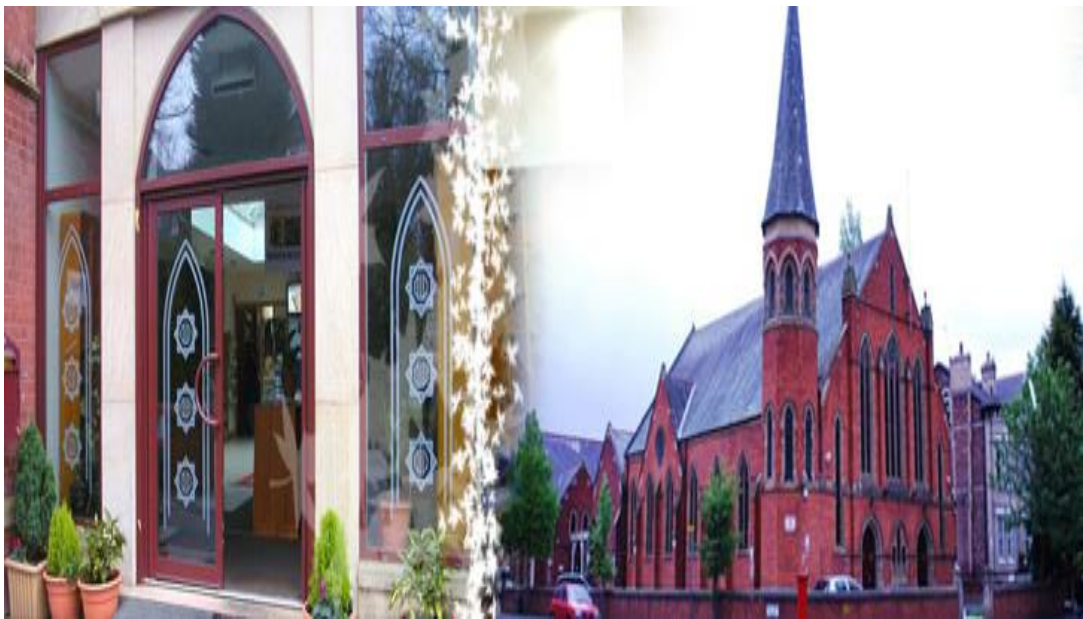
Figure 5.7 Exterior view of Didsbury mosque
