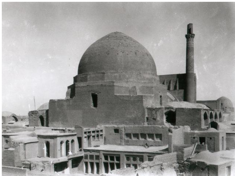
Figure 6.2: The view of the south dome chamber prior to restoration. Taken by Robert Byron 1933-34. ( http://archnet.org/library/images/thumbnails.jsp?location_id=3696 Accessed 10/11/11)
