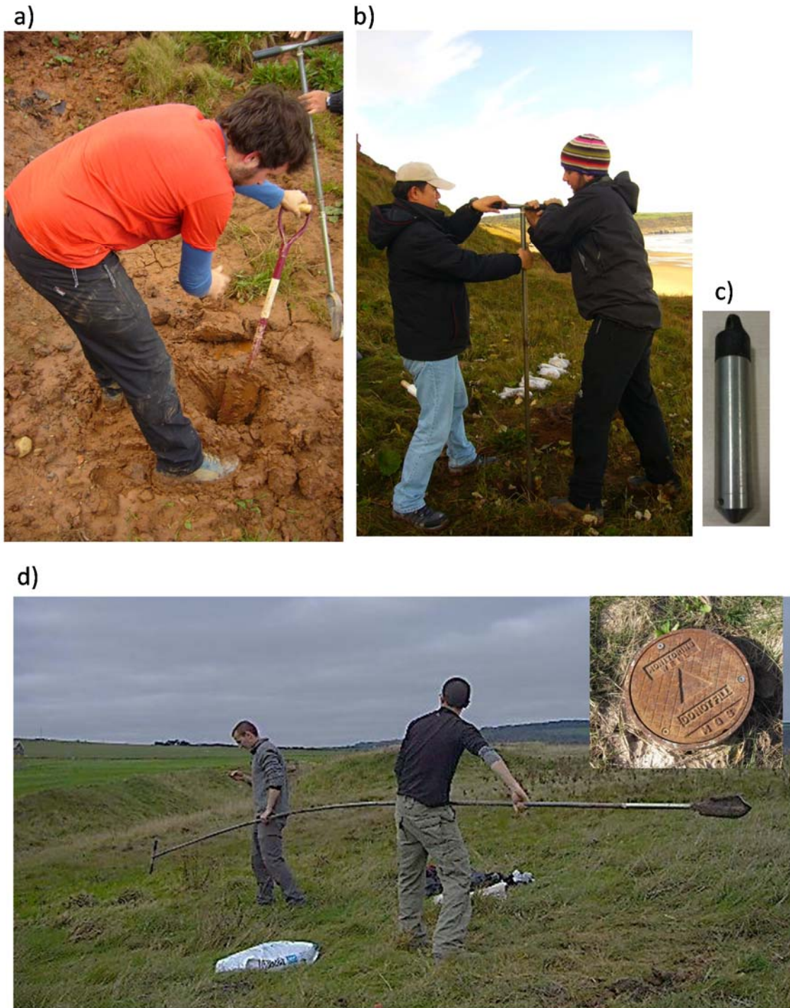
Figure 3.13 Piezometer installation by hand auger: a) preparing the borehole for Casagrande piezometer; b) Using the hand auger to drill a borehole of about 4 inch in diameter; c) Standpipe piezometer tip; d) The long extendable steel rods of hand auger is about 6 m.
