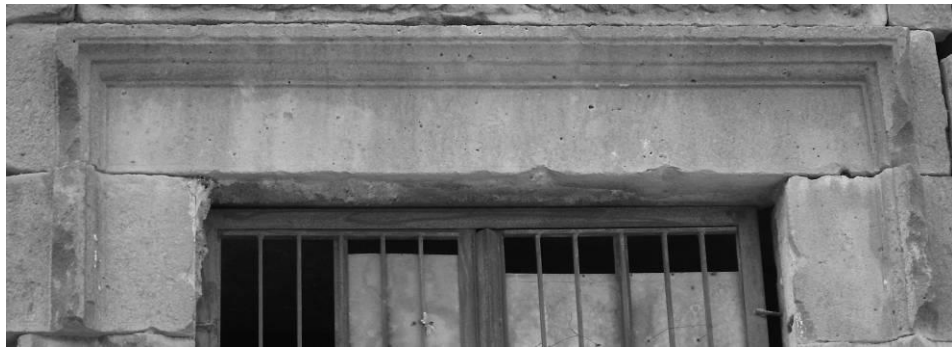
Figure 50: Ionic plain doorframe reemployed in the façade of the sanctuary at Mushannef (by Author 2010)
