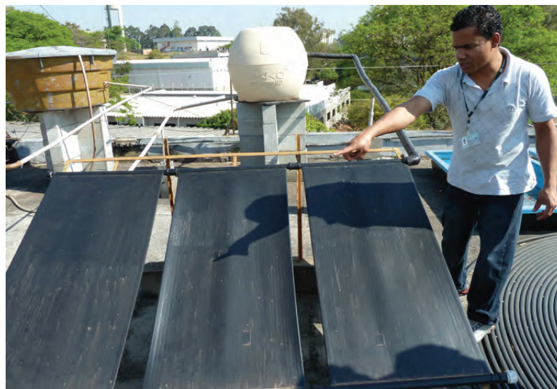
Figure 6.10: DIY SHW system installed at the roof of offices of the Sociedade do Sol , in São Paulo.
