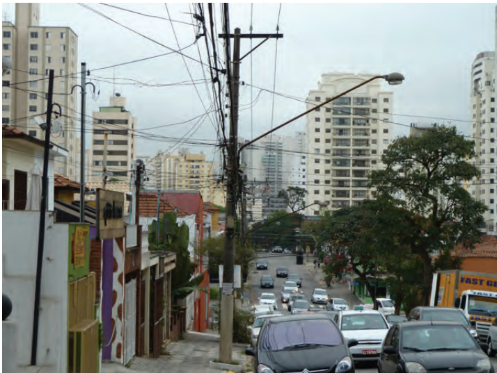
Figure 2.1: Formal electricity provision in central São Paulo
