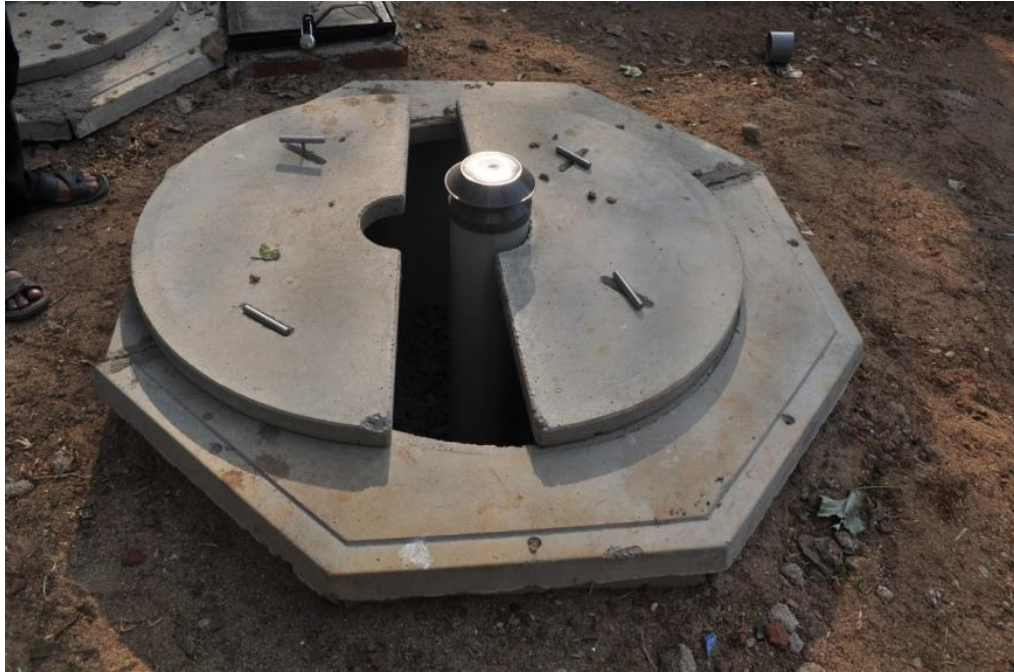
Figure 6.6: Furaat recharge pit and well (Source: Author)
