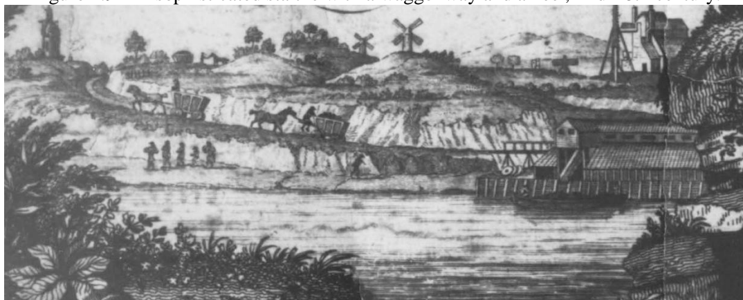
Figure 4.9 – A sophisticated staithe with a waggonway and a keel, mid-18th century.
