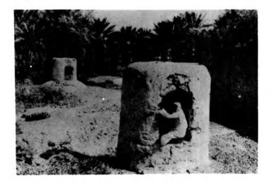
Plate 2.6 Openings along the subterranean canal used for cleaning purposes.
