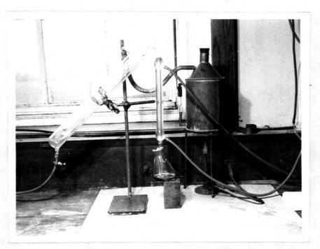
PLATE 9. Markham apparatus for distillation in nitrogen determination.
