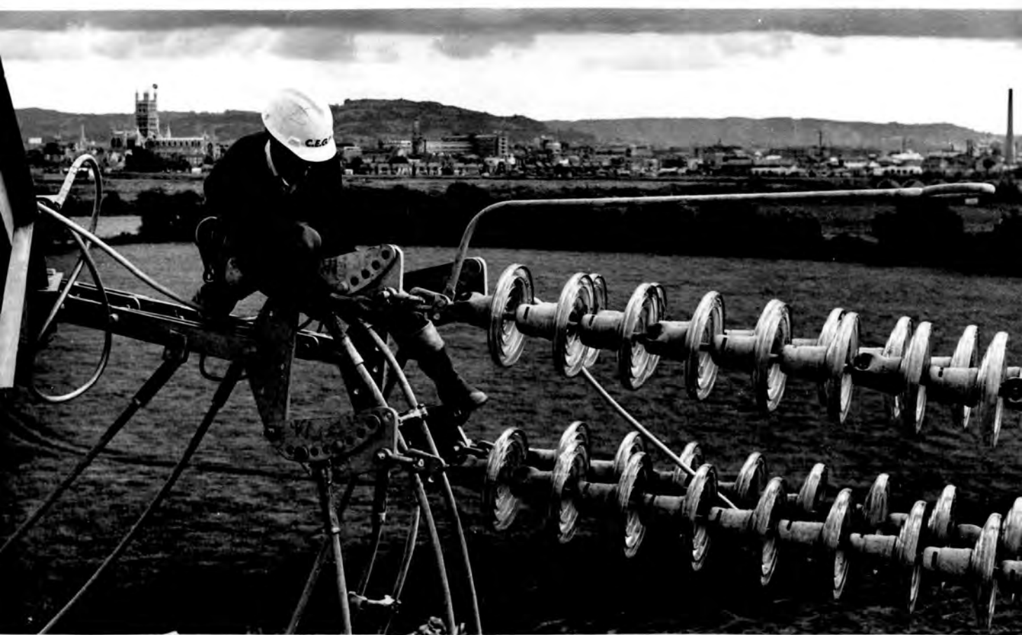
Photograph 66. A tension string of four, 400kV glass insulators, at the Gloucester end of the line to Ystradgynlais substation in South Wales.
