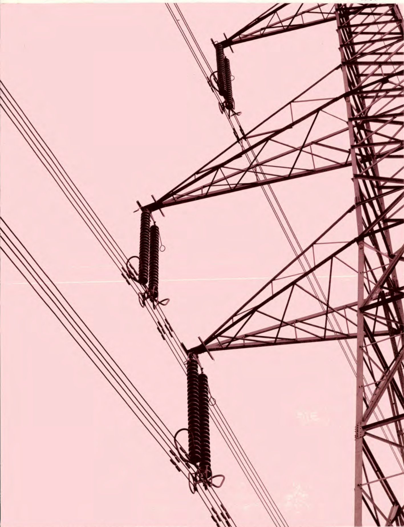
Photograph 63. A 400kV suspension tower showing two strings of porcelain insulators to carry a bundle of four conductors.
