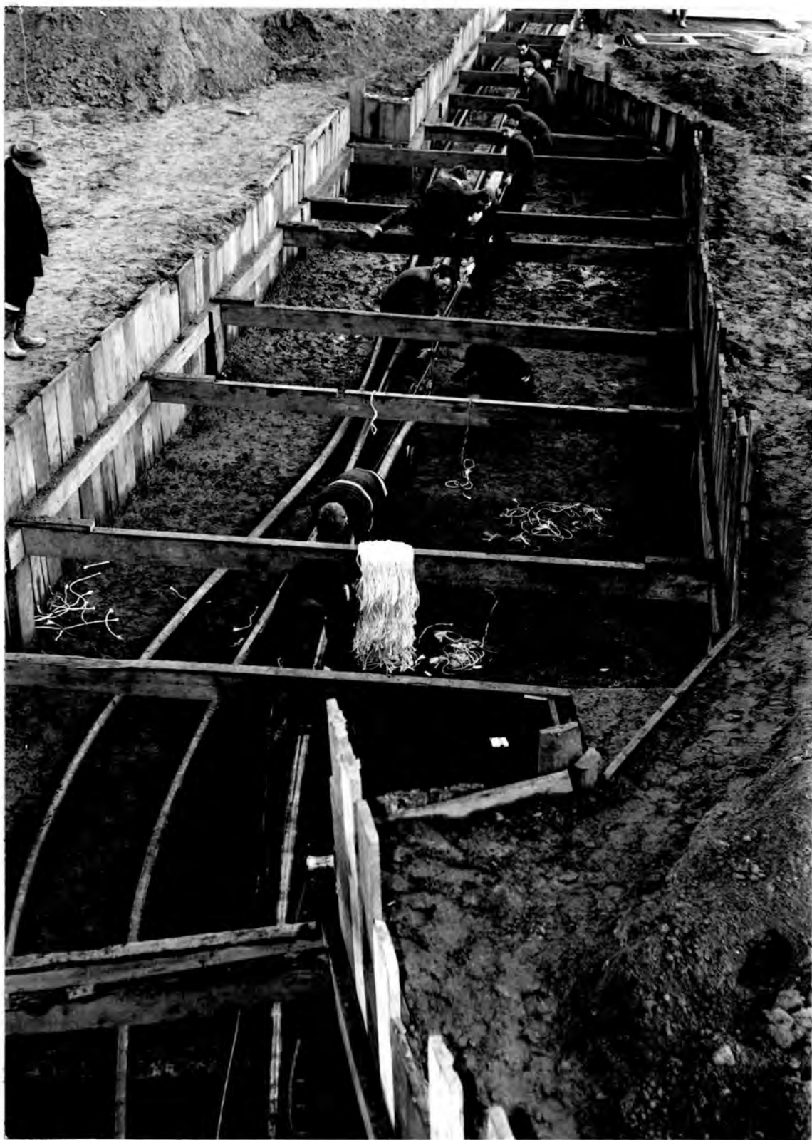
Photograph 29. Shows the width required to join the three phases of one 400 kV cable circuit.
