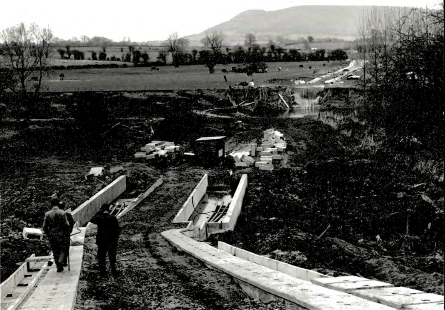
Photograph 35. Installation of concrete troughs for 400 kV cables at approach to the River Wye.
