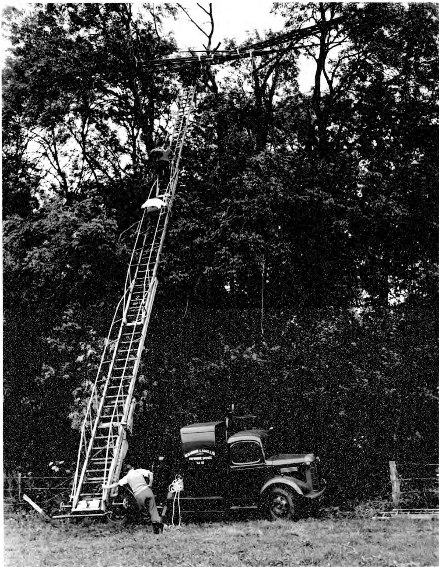
Photograph 22. These trees formed a screen and provided shelter to an orchard in Kent, which required to be crossed by the 275 kV line between Canterbury and Lydd. A fire engine ladder is being used to provide access to the tops of the trees to lash timber poles to carry the conductors during erection to minimise damage, and to avoid felling these trees.
