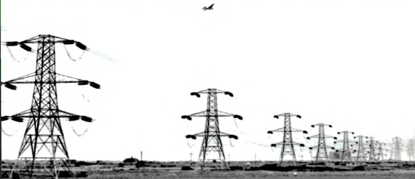
PHOTOGRAPH 8 REDUCED HEIGHT TOWERS CLOSE TOGETHER WITH TENSION INSULATORS. NOTE STANDARD HEIGHT TOWERS TO RIGHT OF PHOTOGRAPH.
