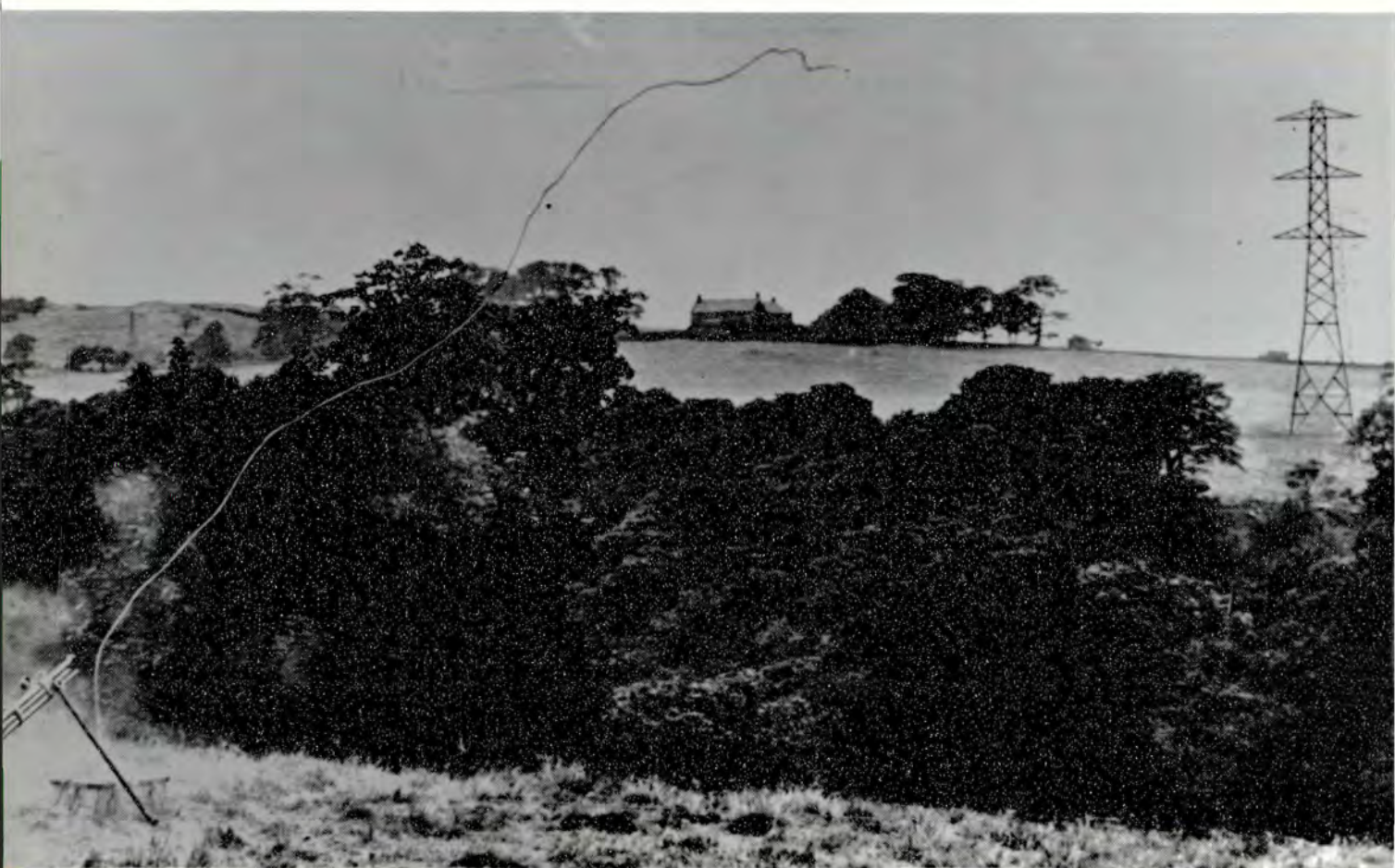
Photograph 23. A rocket carrying a pilot line was used to span the Nant y Ffrith valley, so that conductors could be pulled across without the need to fell the trees.
