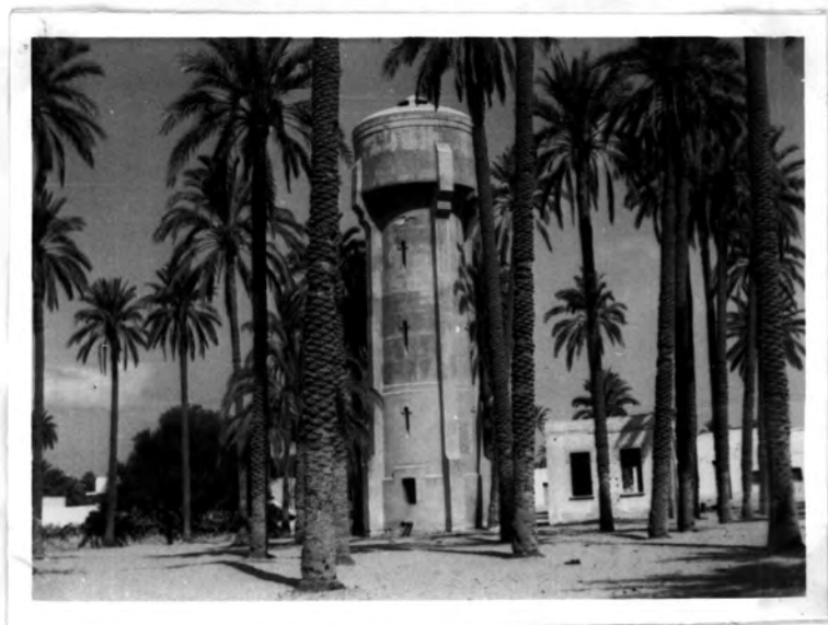
The main water reservoir in Zavla
