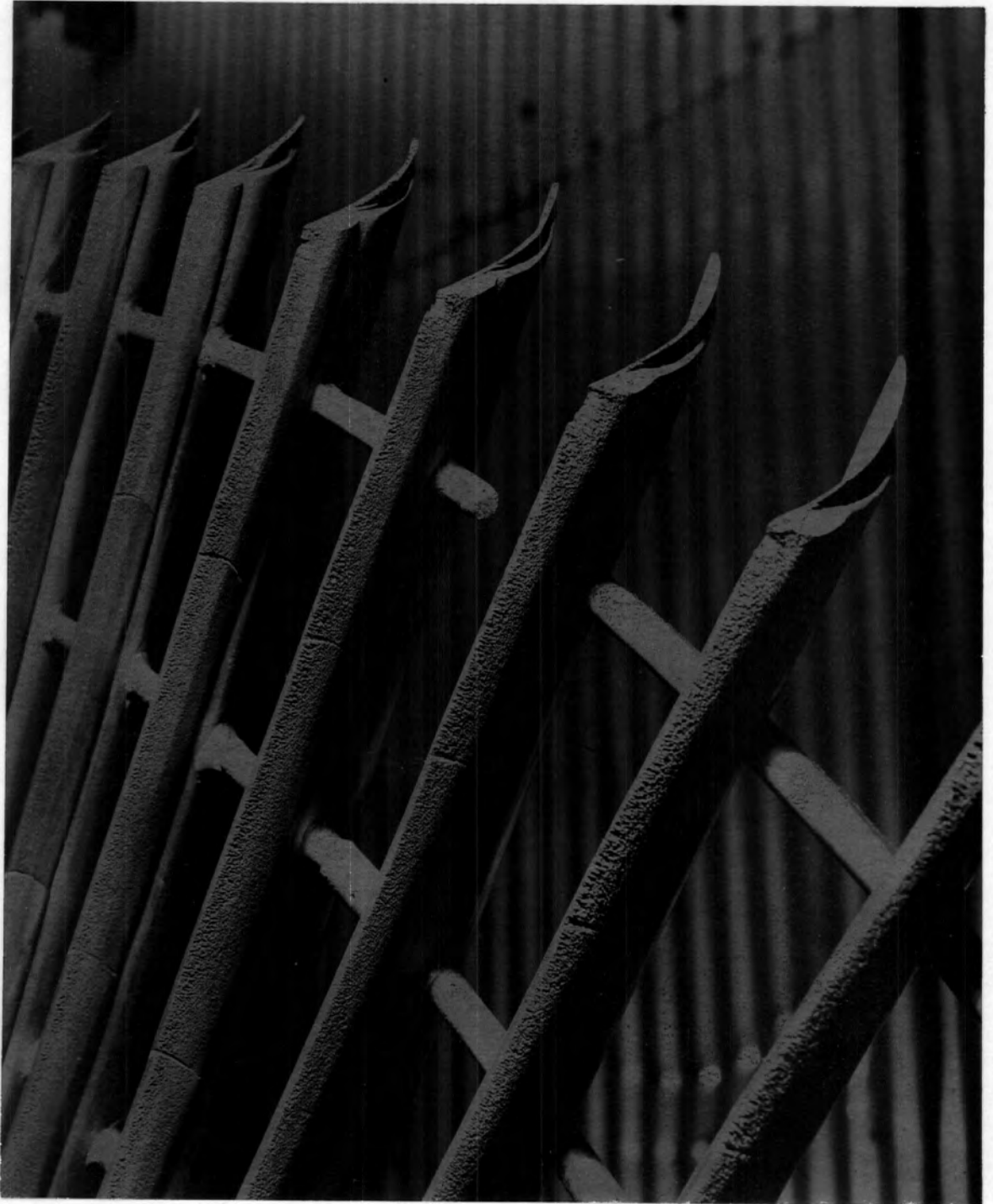
STEAM TURBINE ROTOR ROW SHOWING EROSION DAMAGE TO LEADING EDGE
