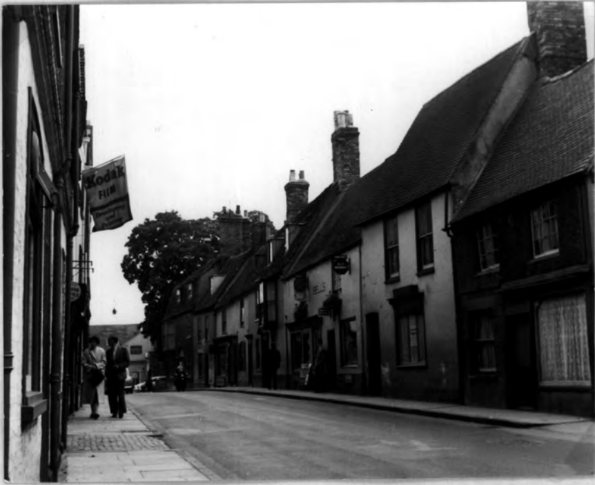
Plate IX. HIGH STREET, looking south towards the river. Old houses, some partly converted into shops.
