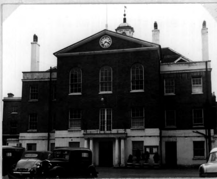
Plate V. TOWN HALL, standing on Market Hill.
