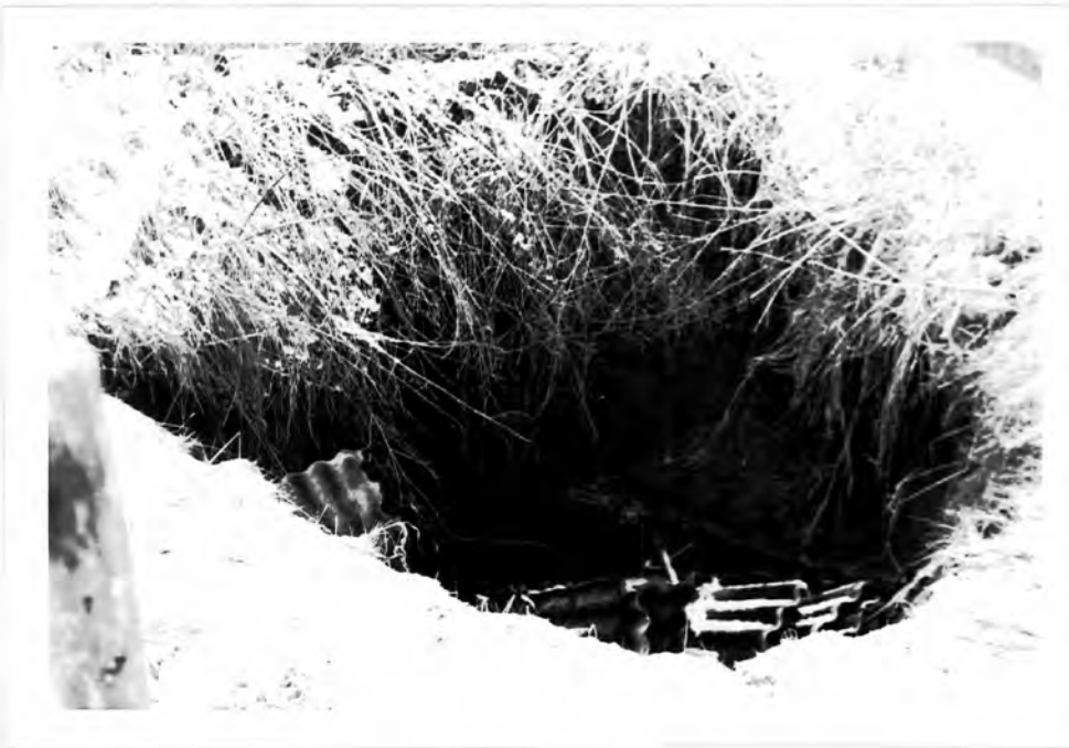
Fig.12. SHAFT KB3. This was probably the shaft worked by the second beam from the engine. It was visible only as an inexplicable diversion in the fence until it caved in in November 1968. It has since been refilled.
